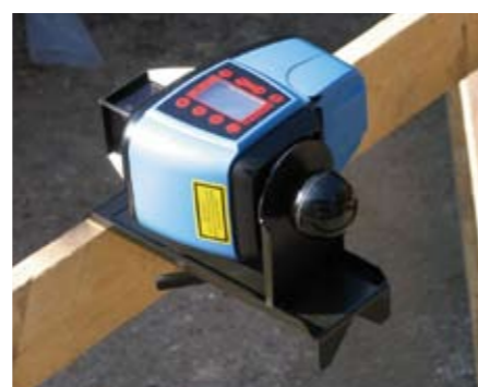
Laser mounted on a batter board
