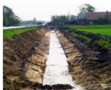
Drainage works and sloping surfaces
